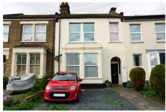
Loss of front garden and boundary for parking, plus uPVC windows and concrete roof tiles
