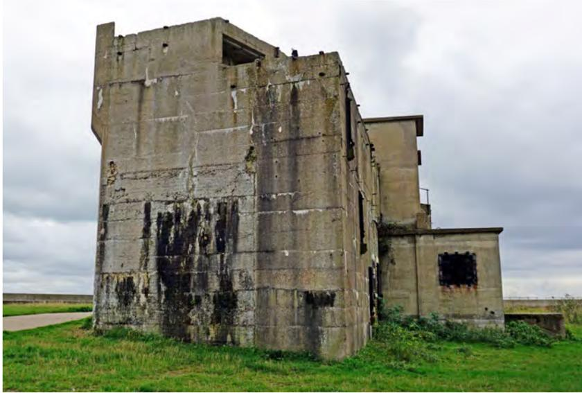
Salt and water staining, and cracked concrete to the Heavy Quick Firing Battery (some remedial work has been carried out to this structure)
